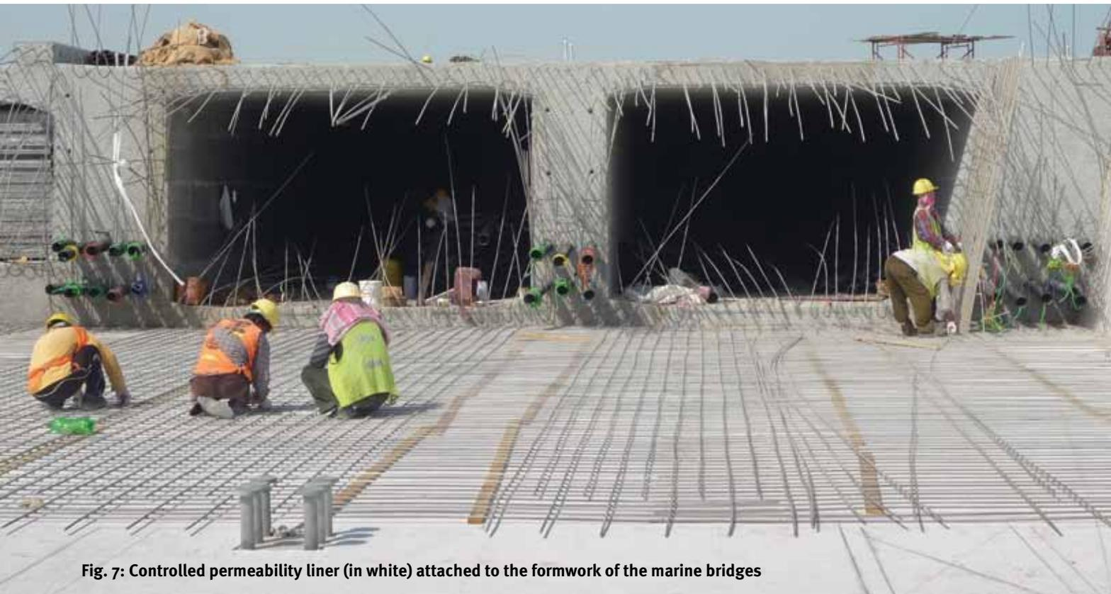
Fig. 7: Controlled permeability liner (in white) attached to the formwork of the marine bridges
