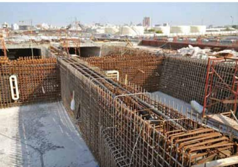
**Fig. 6:** Stainless steel bars were used in the outermost layers of exposed outer and inner surfaces of superstructure elements. Post-tensioning strands were protected using corrugated polyethylene ducts filled with grout
