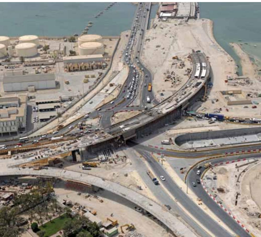
**Fig. 4: Construction of the three-level, grade-separated interchange (looking south)**
