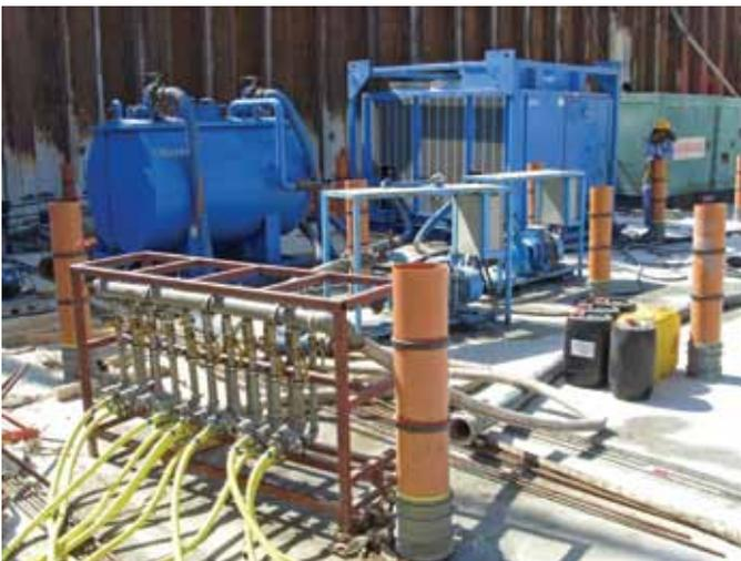
**Fig. 9: Water cooling system (showing chiller, generators, water tank, and control valves)**
