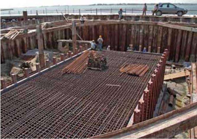
**Fig. 8: Reinforcement cage for a pile cap of a marine bridge pier**
