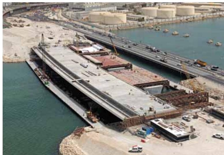
Fig. 2: Completed western carriageway of the northern marine bridge. Temporary staging platforms are in place for the eastern carriageway
