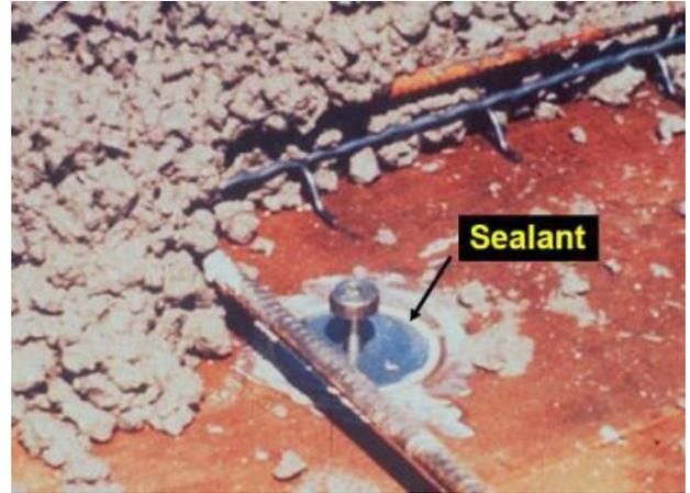
**Figure 11.** LOK bolt in place in floor form
