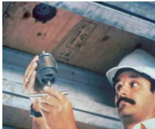
**Figure 12.** Connecting pull bolt to LOK bolt (NOTE: plug removed from porthole)
