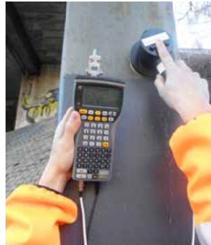
Highway bridge column being tested for corrosion rate with the GalvaPulse
