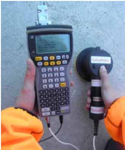
Evaluation of corrosion rate in balcony slab of seaside condominium with the GalvaPulse
