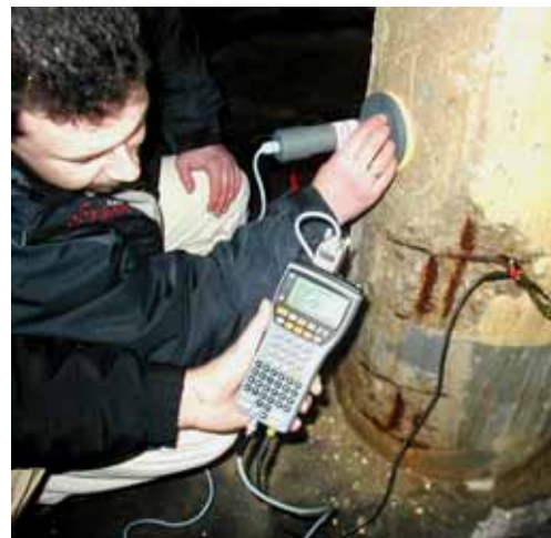
GalvaPulse (older model) testing in progress for corrosion activity of a heavily corroded column
