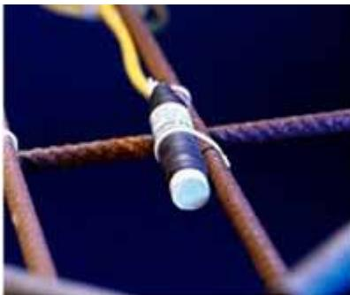
*The **ERE-Probe** attached to reinforcement before placing concrete*
